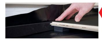
Use spacer blocks to fix the panels 10mm from the wall, or fit the optional plastazote strip.
