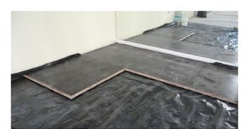
If your room is exactly the same as a row of panels, or the off-cut piece is less than 300mm, then the second row should start using a panel sawn in half.
